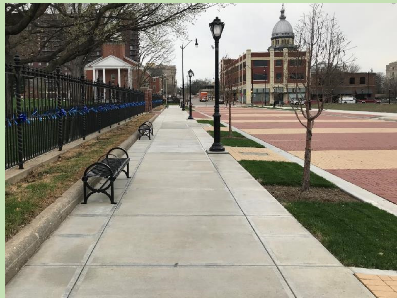
Scored Concrete Sidewalk
