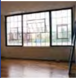
Fig. 15. Original steel windows were retained and made operable during the rehabilitation of this historic mill complex. Insulated sliding windows were added on the interior to improve energy efficiency.
