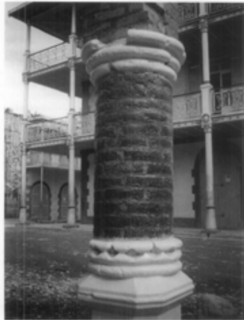
Figure 24. Although the application of a water-repellent coating was probably not needed on either of these buildings, the coating on the brick building (above), is not visible and has not changed the character of the brick. But the coating on the brick column (below), has a high gloss that is incompatible with the historic character of the masonry.
