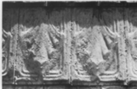
Tin shingles, commonly embossed to imitate wood or tile, or with a decorative design, were popular as an inexpensive, textured roofing material. These shingles 8 1/2 inch by 12 1/2 inch on the exposed surface were designed with interlocking edges, but they have been repaired by surface nailing, which may cause future leakage. (Ballard House, Yorktown, Virginia, photo by Gordie Whitington, National Park Service)
