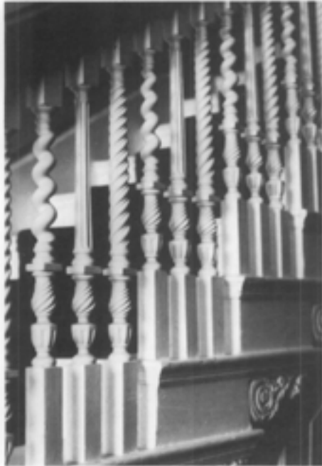
Do not Abrasively Clean these Interiors. Most historic residential and some commercial interior spaces contain finished plaster and wooden elements such as this stair balustrade and paneling which contribute to the historic and architectural character of the structure. Such interiors should not be subjected to abrasive techniques for the purpose of removing paint, dirt, discoloration or plaster.
