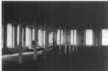
Permissible Abrasive Cleaning. In accordance with the Secretary of the Interior's Guidelines for Rehabilitation Projects, it may be acceptable to use abrasive techniques to clean an industrial interior space such as that illustrated here, because the masonry surfaces do not have significant design, detailing, tooling or finish, and the wooden architectural features are not finished, molded, beaded or worked by hand.
