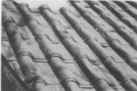
Galvanized sheet-metal shingles imitating the appearance of pantiles remained popular from the second half of the 19th century into the 20th century. (Episcopal Church, now the Jerome Historical Society Building, Jerome, Arizona, 1927)
