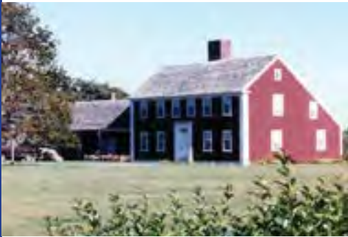
Fig. 4. A typical New England saltbox features a steeply sloping roof to shed snow and a floor plan organized around a central chimney to conserve heat.
