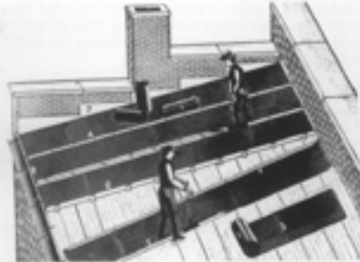
A Chicago firm's catalog dated 1896 illustrates a method of unrolling, turning the edges, and finishing the standing seam on a metal roof.
