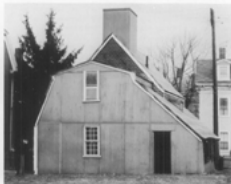
Temporary stabilization or "mothballing" with materials such as plywood and building paper can protect the roof of a project until it can be properly repaired or replaced. (Narbonne House, Salem, Massachusetts)
