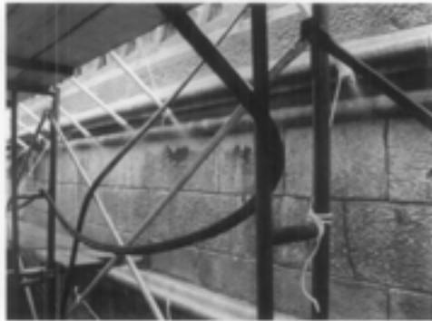
Figure 6. Timed water soaking can be very effective for cleaning limestone and marble as shown here at the Marble Collegiate Church in New York City. In this case, a twelve-hour water soak using a multi-nozzle manifold was followed by a final water rinse. Photo: Diane S. Kaese, Wiss, Janney, Elstner Associates, Inc., N.Y., N.Y.
