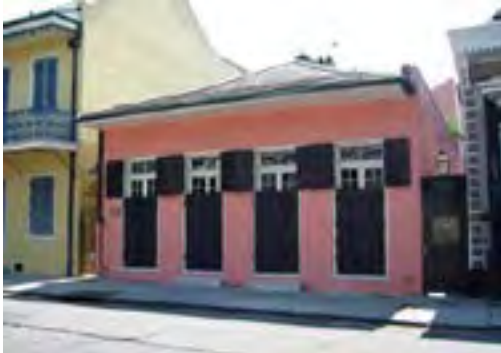
Fig. 2. Upper and lower shutters control daylight and provide privacy.
