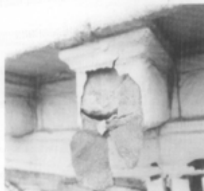
Figure 27. Instead of correcting the roof drainage problems, an elastomeric coating was applied to the already saturated limestone cornice. An elastomeric coating holds moisture in the masonry because it does not "breathe" and does not allow liquid moisture to escape. If the water pressure builds up sufficiently it can cause the coating to break and pop off as shown in this example, often pulling pieces of the masonry with it. Photo: National Park Service Files.
