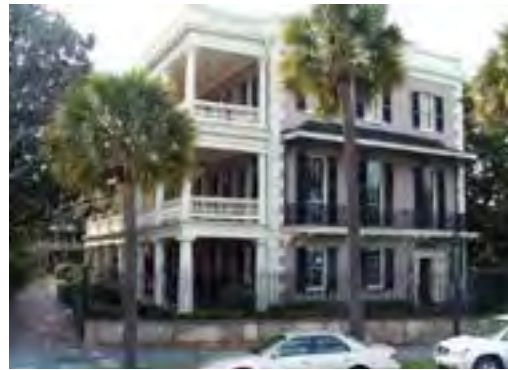
Fig. 5. The side porches of this house in Charleston, SC, shade the large windows and provide outdoor living spaces that take advantage of sea breezes.
