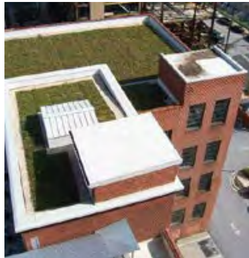
Fig. 22. Installation of both cool and green roofs in an urban environment.
