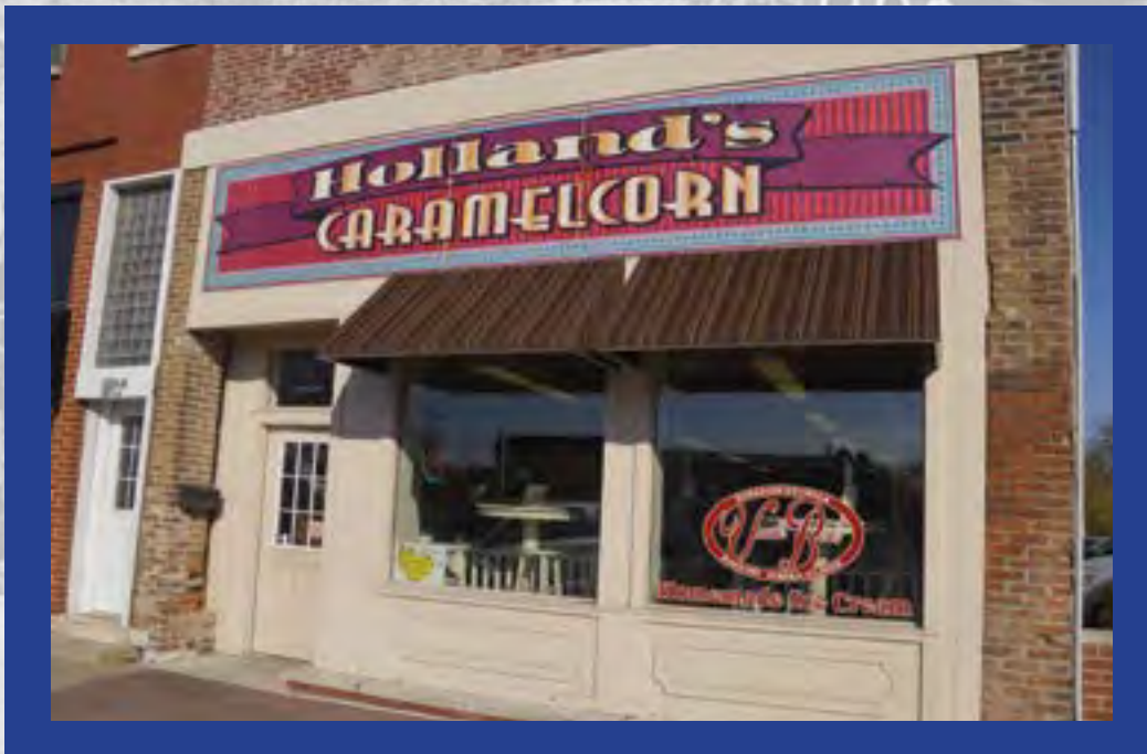
A variety of types of entrances are used around the Square; here, Holland's provides an accessible entrance with no step in front.
