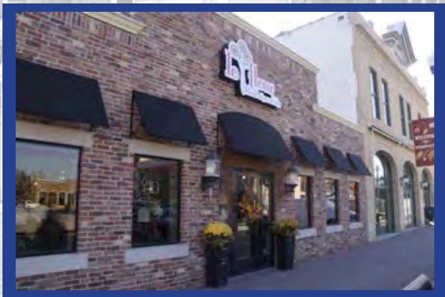
There are a variety of styles of awnings throughout the Square; le Fleur uses fixed individual awnings on their storefront.
