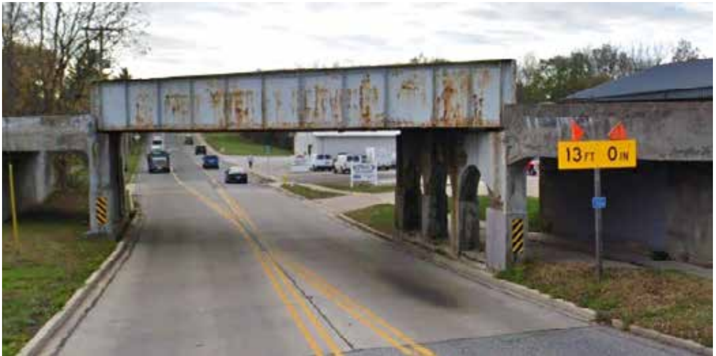
Figure 3: Toledo Peoria/Western Railway Bridge Crossing
